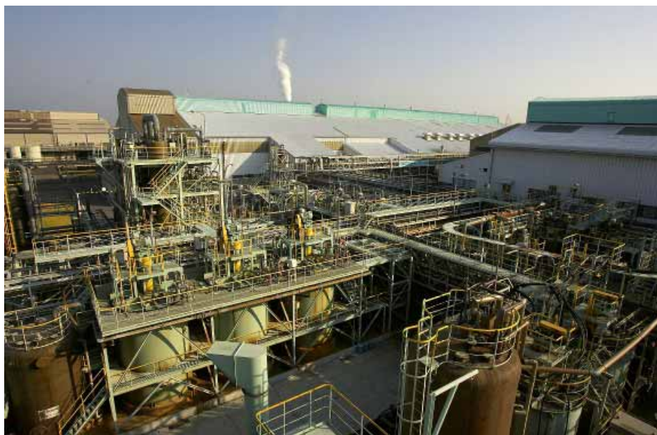
Niihama Nickel Refinery
