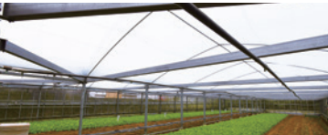
Greenhouse with a roof tent woven with fibers of dispersed near-infrared absorbing material of cesium tungsten oxide (CWO*)
