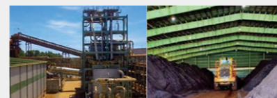
Chromite production facility and storage area
