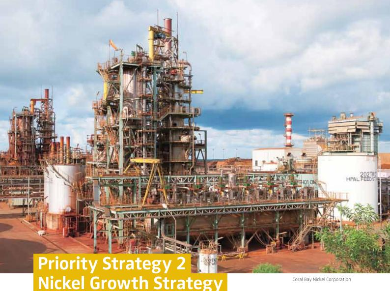
SMM has an undisputed strength in nickel operations. That is our success in being the first company in the world to effectively use High Pressure Acid Leach (HPAL) technology on a commercial basis. With this technology, it is possible to recover nickel from low-grade ore. Consequently, even in an environment marked by declines in nickel resources, the Company will be able to steadily secure raw materials at low cost and expand its nickel operations.
